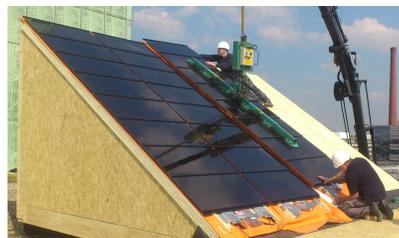
**Figure 7** Crane mounting the prototype roof insulation integrated PV elements on the constructed artificial test roof in May 2014.
