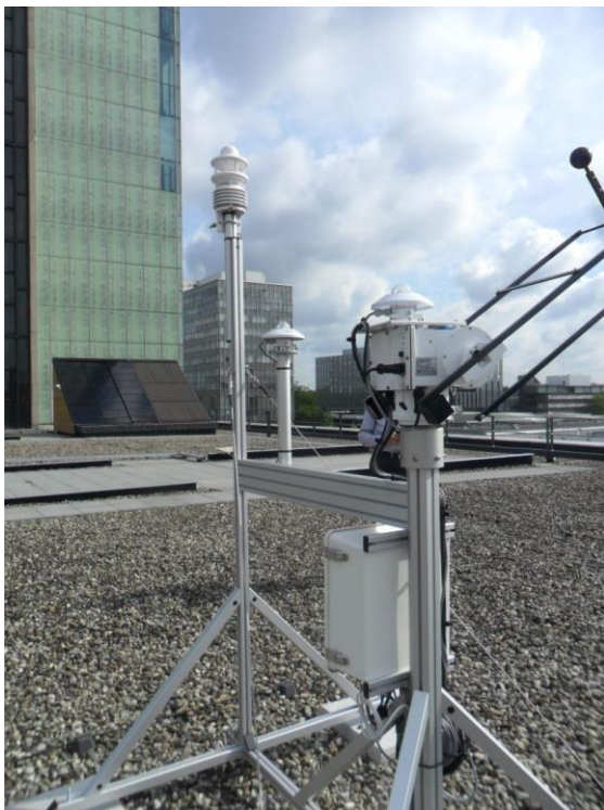
Figure 2: Solar Measurement and Weather Station at SolarBEAT. The green building in the background is in the North.
