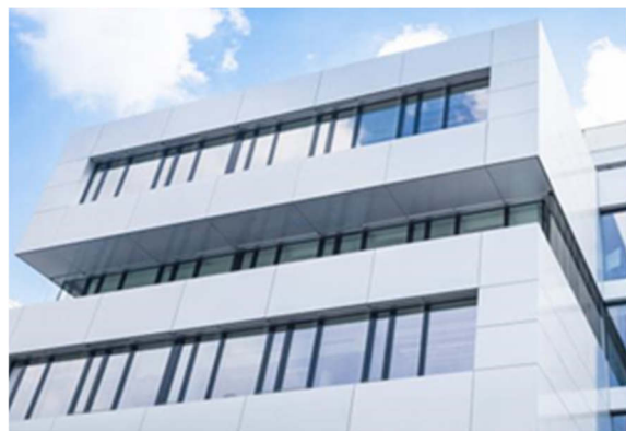
Figure 3: A BIPV white module obtained through a laminated color foil with diffuse reflector (Solaxess).
