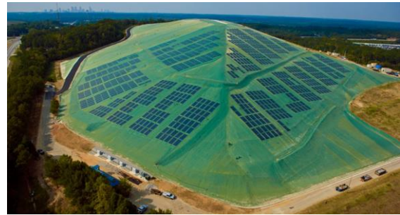
Figure 4. PV integrated geomembrane at the Hickory Ridge landfill in Georgia
