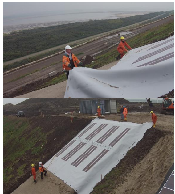
Figure 5. Installation of the exposed geo-membrane solar capping phase I
