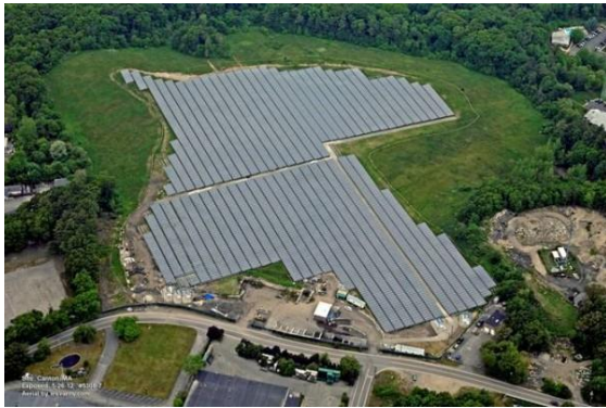
Figure 2. Aerial view of 5.75 MW Ground-Mounted Solar System installed on the Canton landfill, Massachusetts
