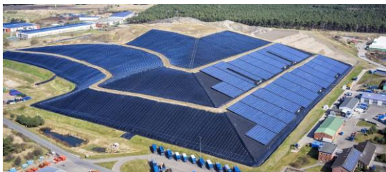
Figure 3. 3.8MWp PV system in Lunenburg landfill
